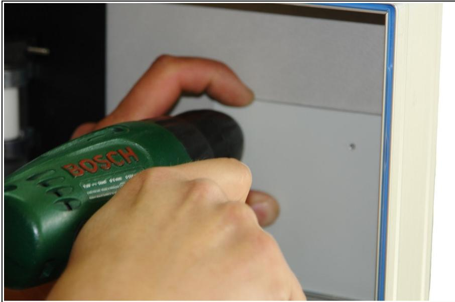
Picture 4. Drilling the holes in the cover with the help of the stencil.
